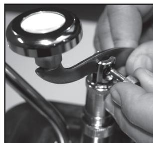
(Photo 1) Unscrew set screw and remove lever.
